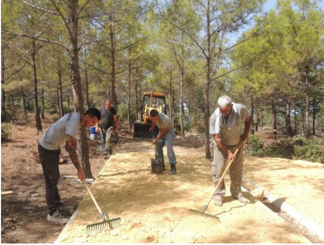
Fig 21: Building Process of the Walking Path (Municipality Website)
